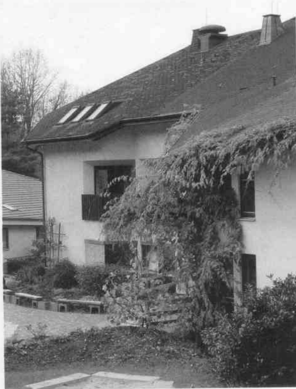
Fig. 13: ►► HAUS TOBIAS: LAUNDRY WASHED WITH RAINWATER
