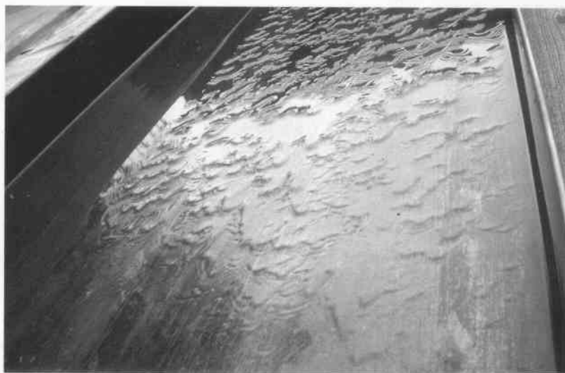
Fig. 9+10: BRUCKFELDEN SCHOOL: U-SHAPED OPEN DOWN PIPE
