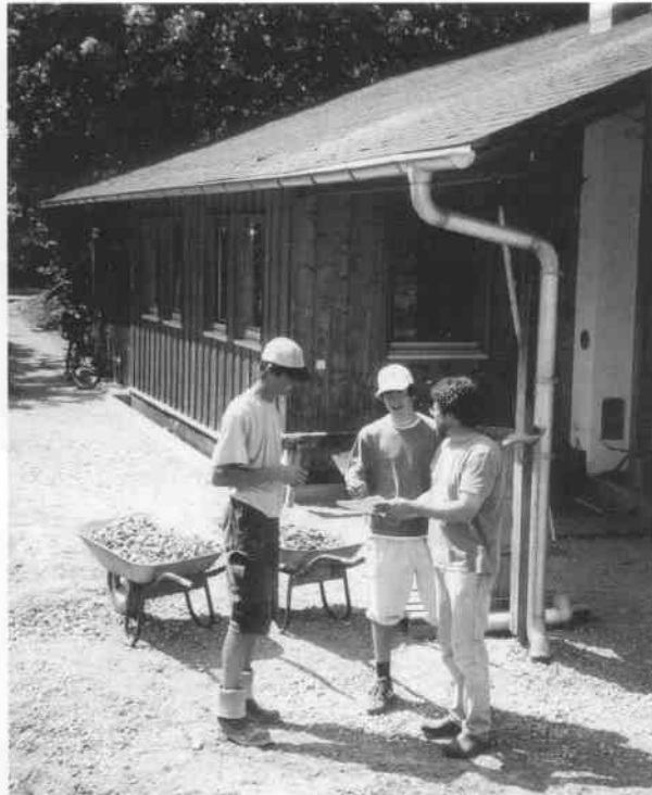
Fig. 6: STEINER SCHOOL: STUDENT BUILDING IRRIGATION SYSTEM WITH RAINWATER
