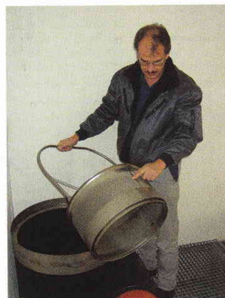
Figure 3: Rainwater filter – removal of vortex fine filter device to be cleaned (Photo: Klaus W. König)
