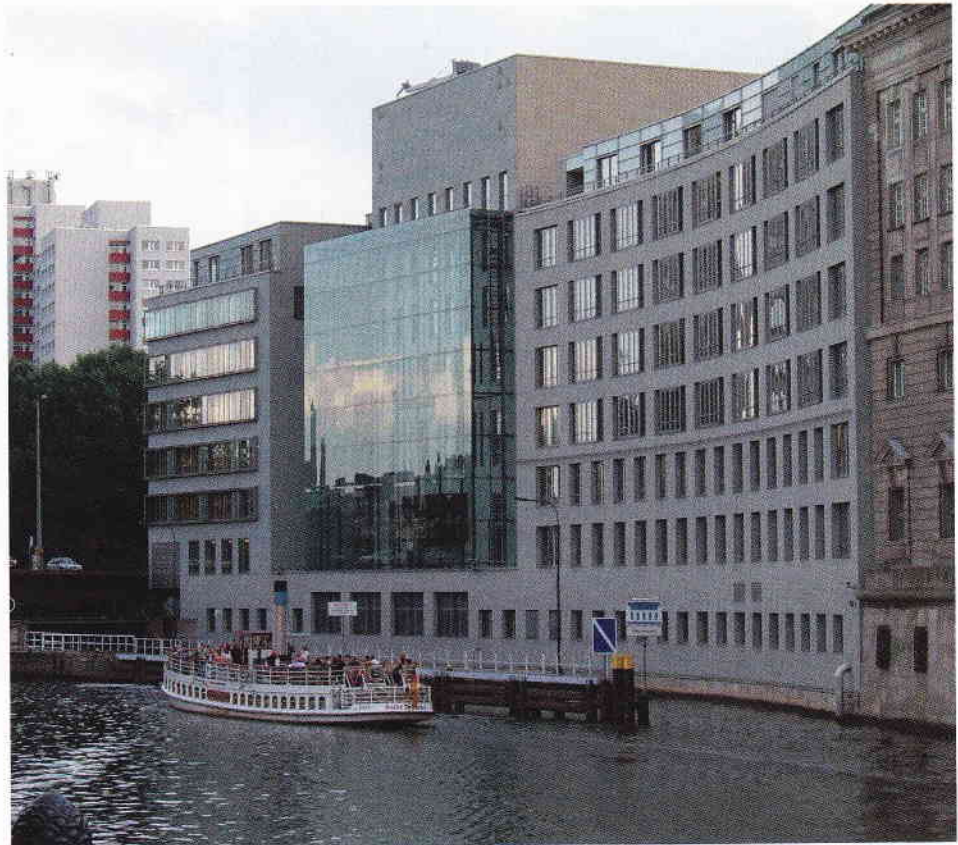
Figure 8: View of building from River Spree. Overflow of rainwater system in bottom right of picture -stainless steel pipe. (Photo: Klaus W. König)
