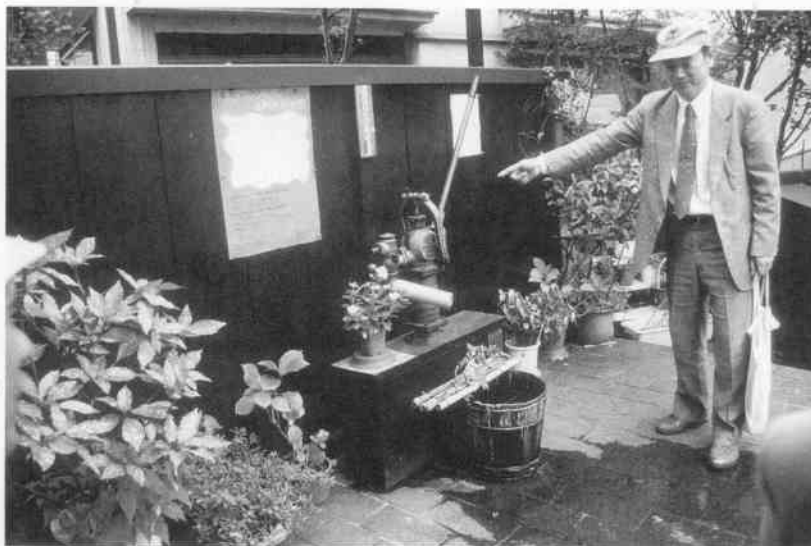
Fig. 2 ROJISON IS A RAIN WATER TANK WHICH IS ACCESSIBLE FOR THE PUBLIC IN THE MATTER OF A DISASTER
