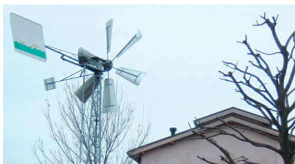
Fig. 7. Wind turbine, power generation for supply of the rainwater circulation pump for the biotope and open water. Photo: König
