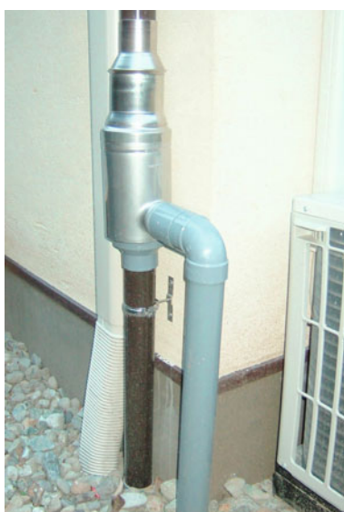
Fig. 3. Rainwater filter made in Germany, Wisy down pipe filter SAGF type at the rainwater down pipe. Photo: König
