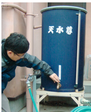
Fig. 6. Rainwater reservoir above ground installed for easy access by children for irrigation purposes. Photo: König
